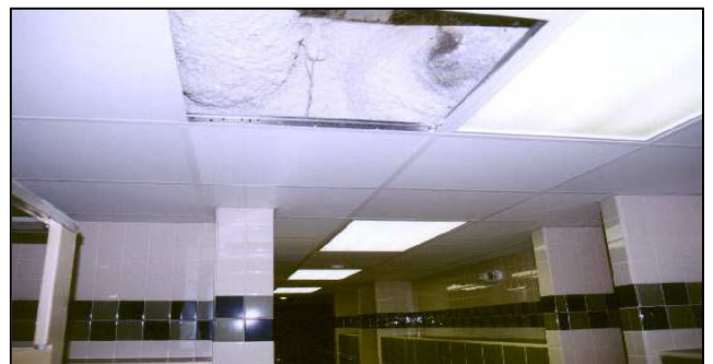
Underside of Patio – Locker Room
